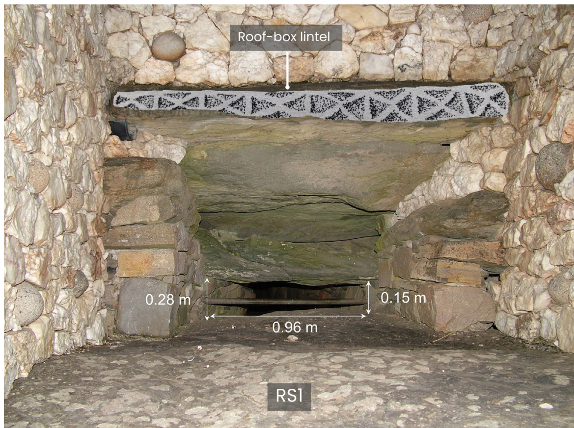
Figure 6: Newgrange roof-box looking into the tomb. (Photo and roof-box dimensions are by F Prendergast with an overlay of the lintel decoration from a drawing by Claire O’Kelly, 1973).
